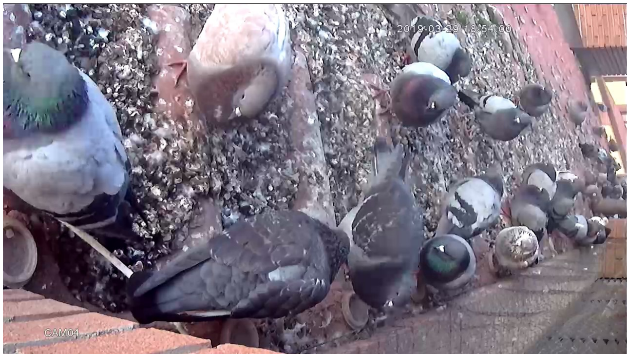
Figure 21. North roof two years after the installation with Empty Dishes
