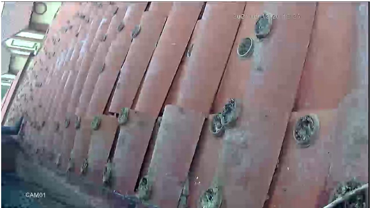
Figure 22. South roof four years after BIRD FREE installation
