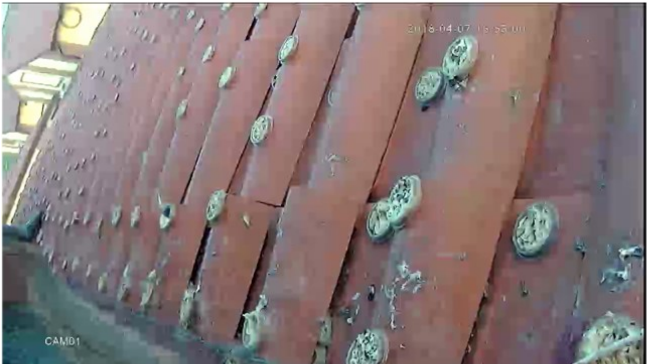
Figure 18. South Roof provided with BIRD FREE . The picture has been taken at the sunset after about 1 year from the installation.
