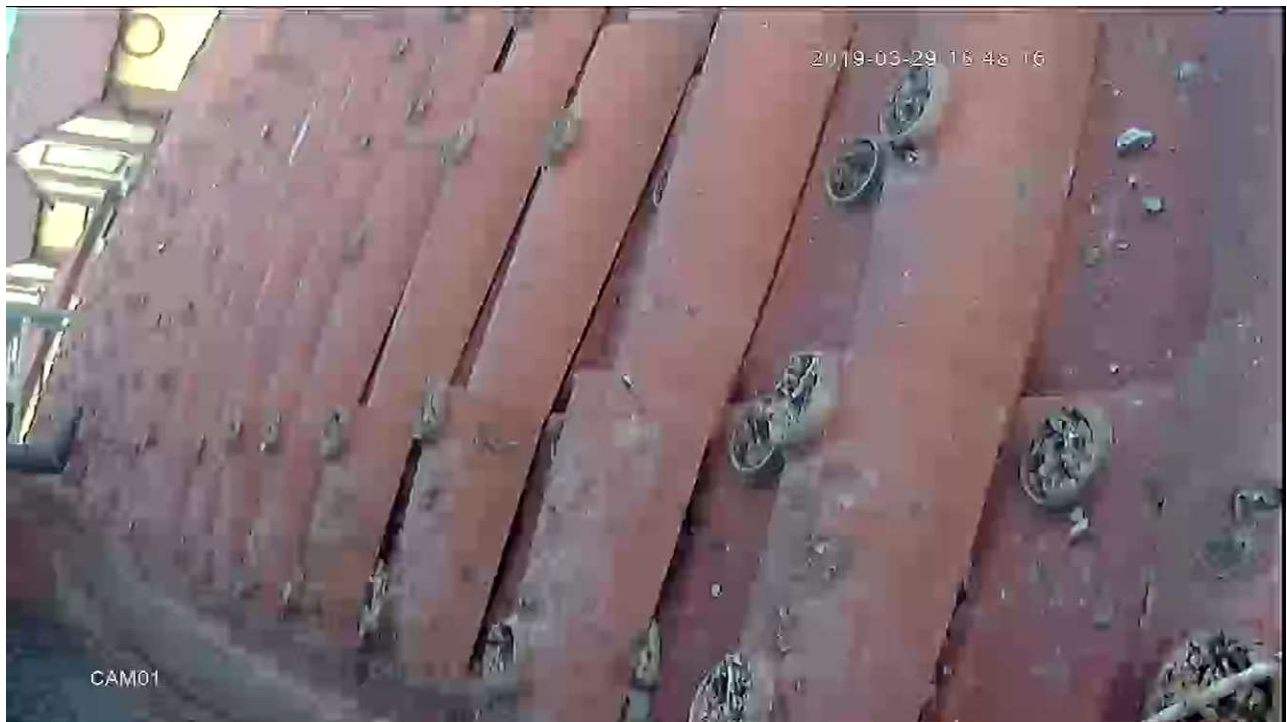
Figure 20. South roof two years after BIRD FREE installation
