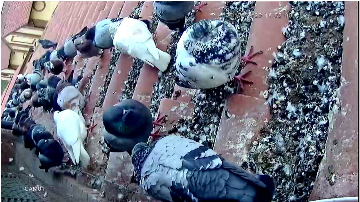
Figure 5. Picture of the South Roof taken on the 26 th of March 2017 before the sunset (18:33), three days before the installation of BIRD FREE .
