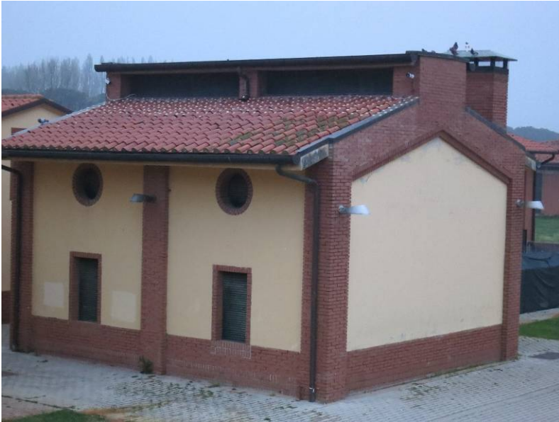
Figure 9. South roof after the installation of BIRD FREE
