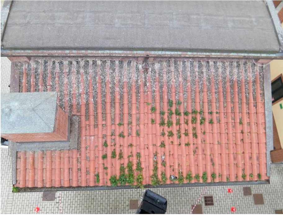
Figure 11. North Roof before the treatment.
