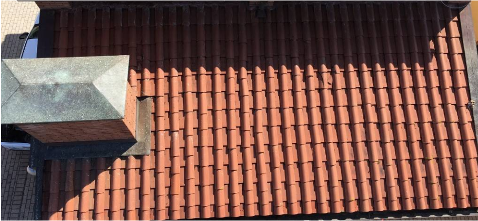
Figure 13. North roof cleaned and disinfected.
