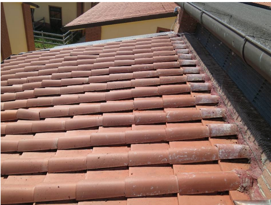
Figure 6. South roof after bird dropping removal and cleaning.
